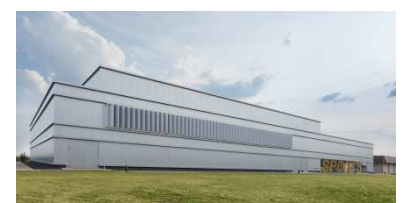
Neubau Physical Fitness Center, Katterbach
